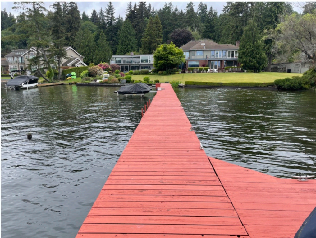
Photo 2 - Existing dock looking landward.
