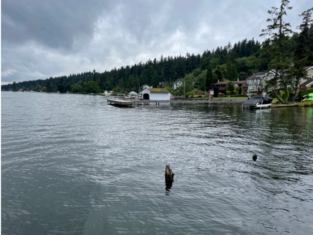
Photo 5 - Shoreline conditions south of the site. Note broken mooring piles to be removed.
